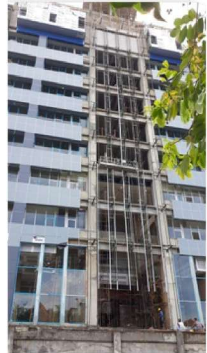
Steel frame facade
