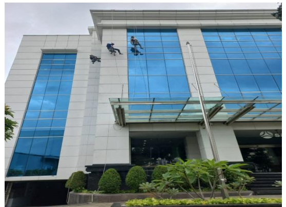
Painting with Rope Access For High Level Building
