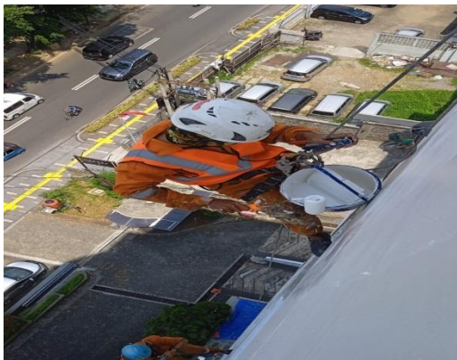
Painting with Rope Access For High Level Building
